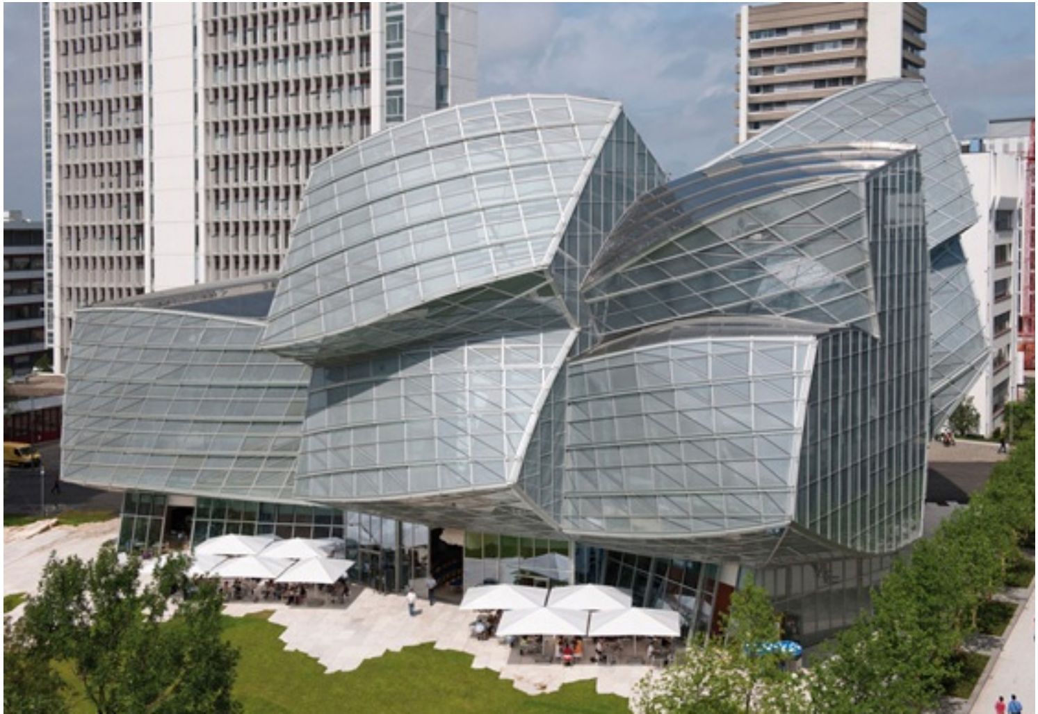
Innovative Photovoltaik GEHRY BUILDING NEW YORK © sunways.de
